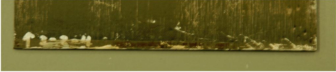
Figure 5.16: Close up view of the burned surface on sample 3-2-4
